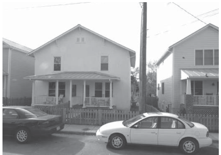
6. Anderson Street Home with new residences, creating a denser fabric of street-facing homes. The house in the middle is an image after renovation and construction of the new houses; the older home is located in the middle. (Photo by Will Kerner, 2006)
