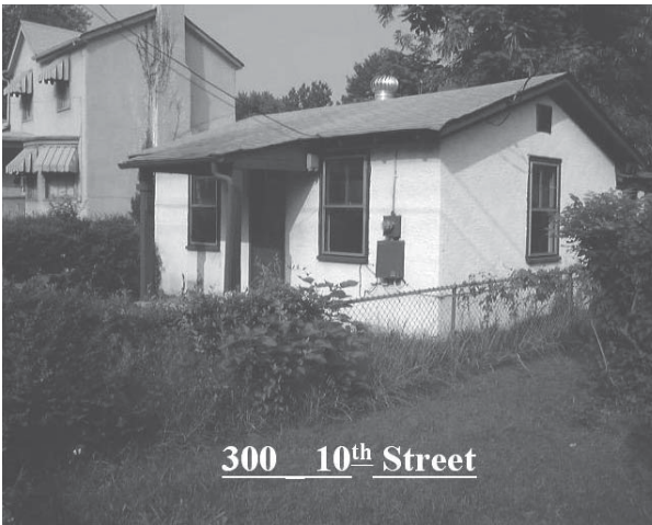
3. One of the 10th street slab-on-grade houses. (Photo by PHA, 2000)
