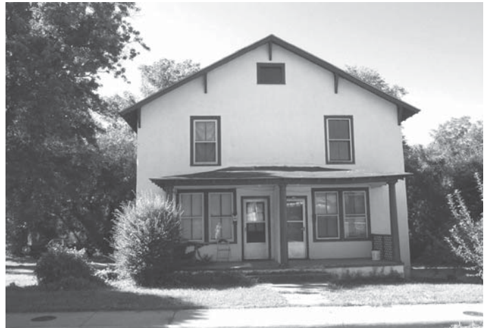
5. House on Anderson Street before renovation (Photo by Author, 2000)
