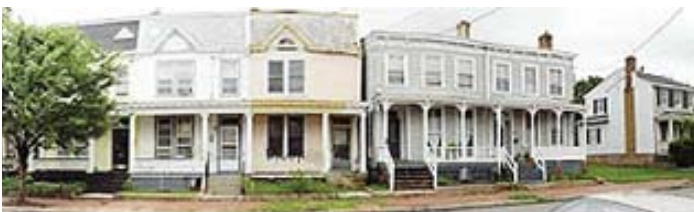
9. The Richmond, Virginia Neighborhood of Church Hill Central, One of the Six "Neighborhoods in Bloom" Areas, www.ci.richmond.va.us/departments/communityDev/neighborhoods
