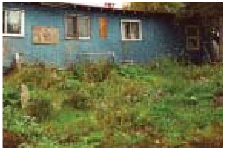
The widow who occupies this home is struggling against deterioration and air infiltration as the unit fails to provide her in her old age with the secure housing envisioned by her and her husband when they purchased it 30 years ago.
