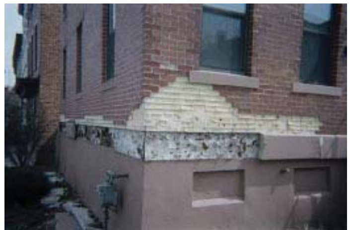
Designers and developers have insufficient resources to evaluate the longevity of materials as evidenced by the decay of this 17-year-old affordable infill housing.
