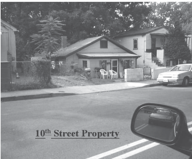
The preservation community was understandably alarmed at the loss 4. House slated for demolition showing the site and material conditions (photo by PHA, 2000).
