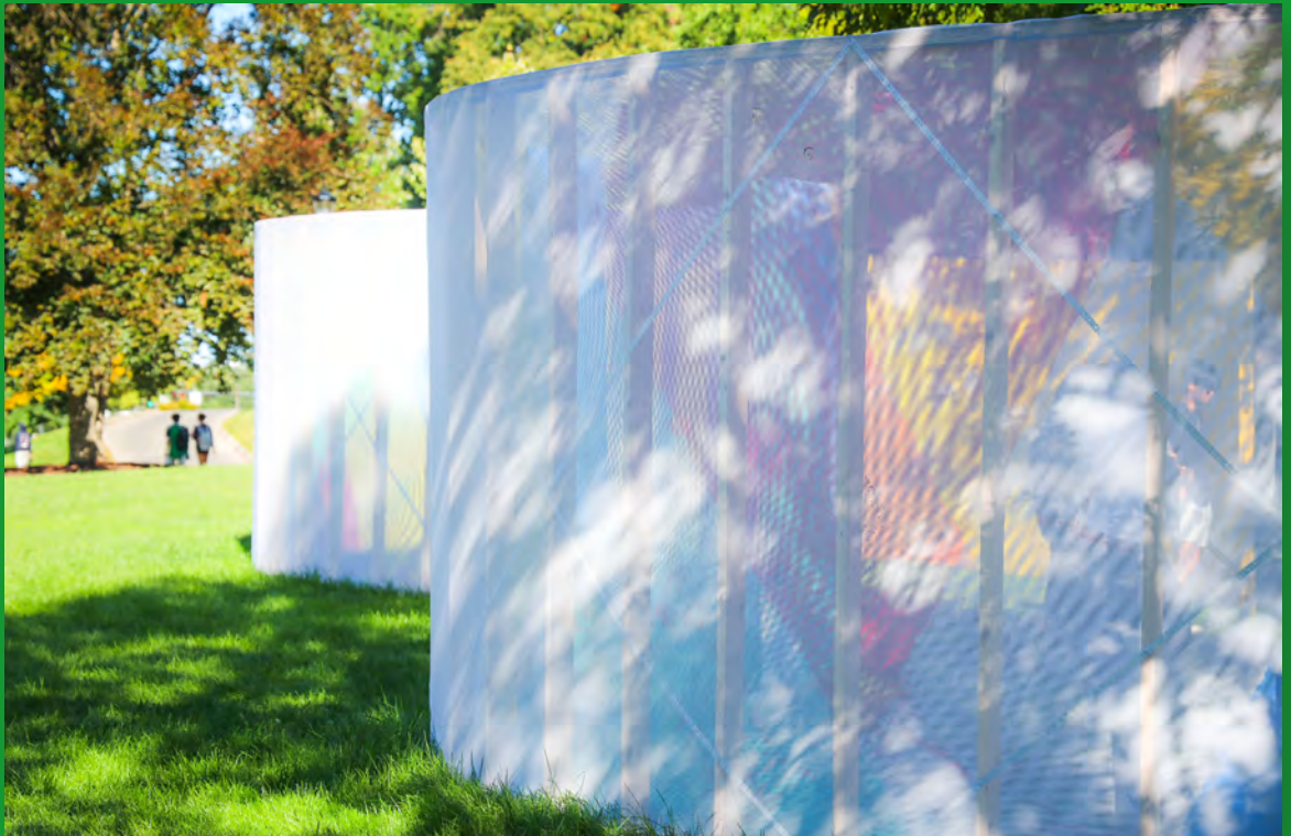
Above: STEP high schools students building the structural walls of the pavilion on campus. Below: Cornell classes being held in the pavilion (visible through the translucent skin).
