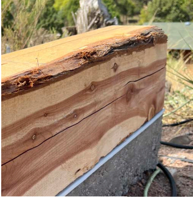
First course laid
