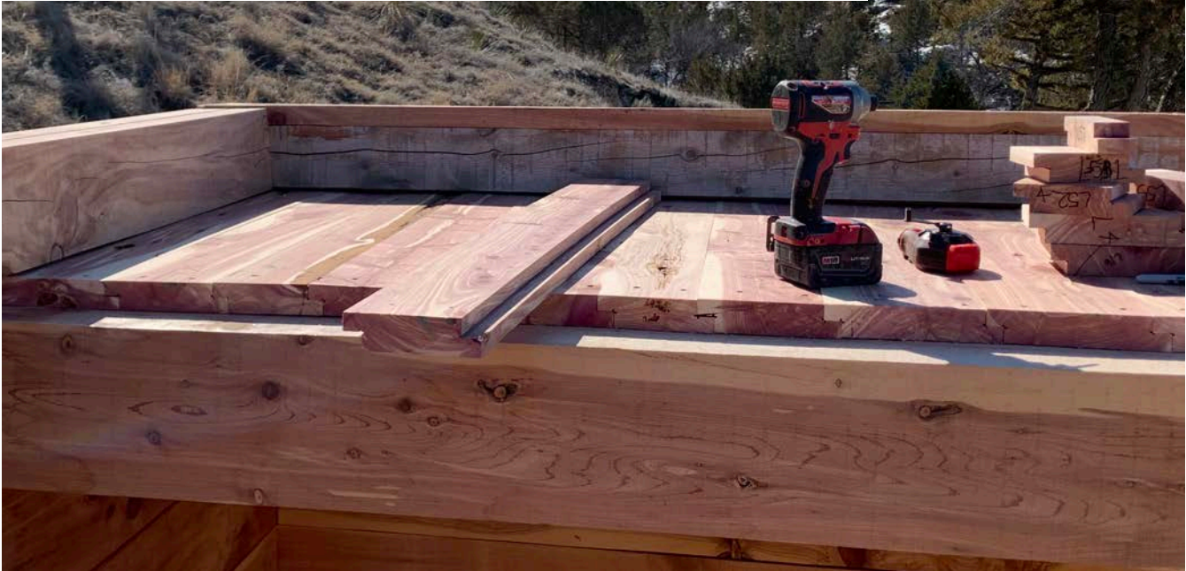
Half lap cedar roof deck Installation
