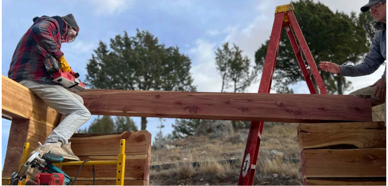
Lintel course laid
