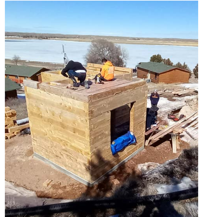
Wall assemblies completed
