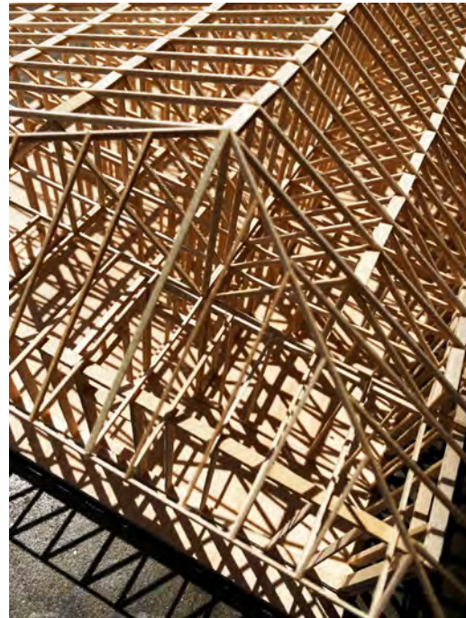
ABOVE: studies of construction material technologies and their impact on time and cost were studied during the design process of Timberlands Prototype 01; BELOW: framing model of the traditional stick-built construction strategy chosen for the initial prototype
