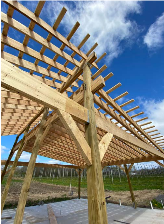
Figure 2. Structural Framing. Photograph by author.
