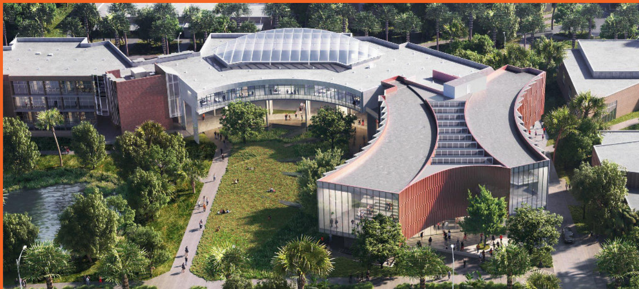
Bruno E. and Maritza F. Ramos Collaboratory, 2025 Addition to the University of Florida Architecture Building
