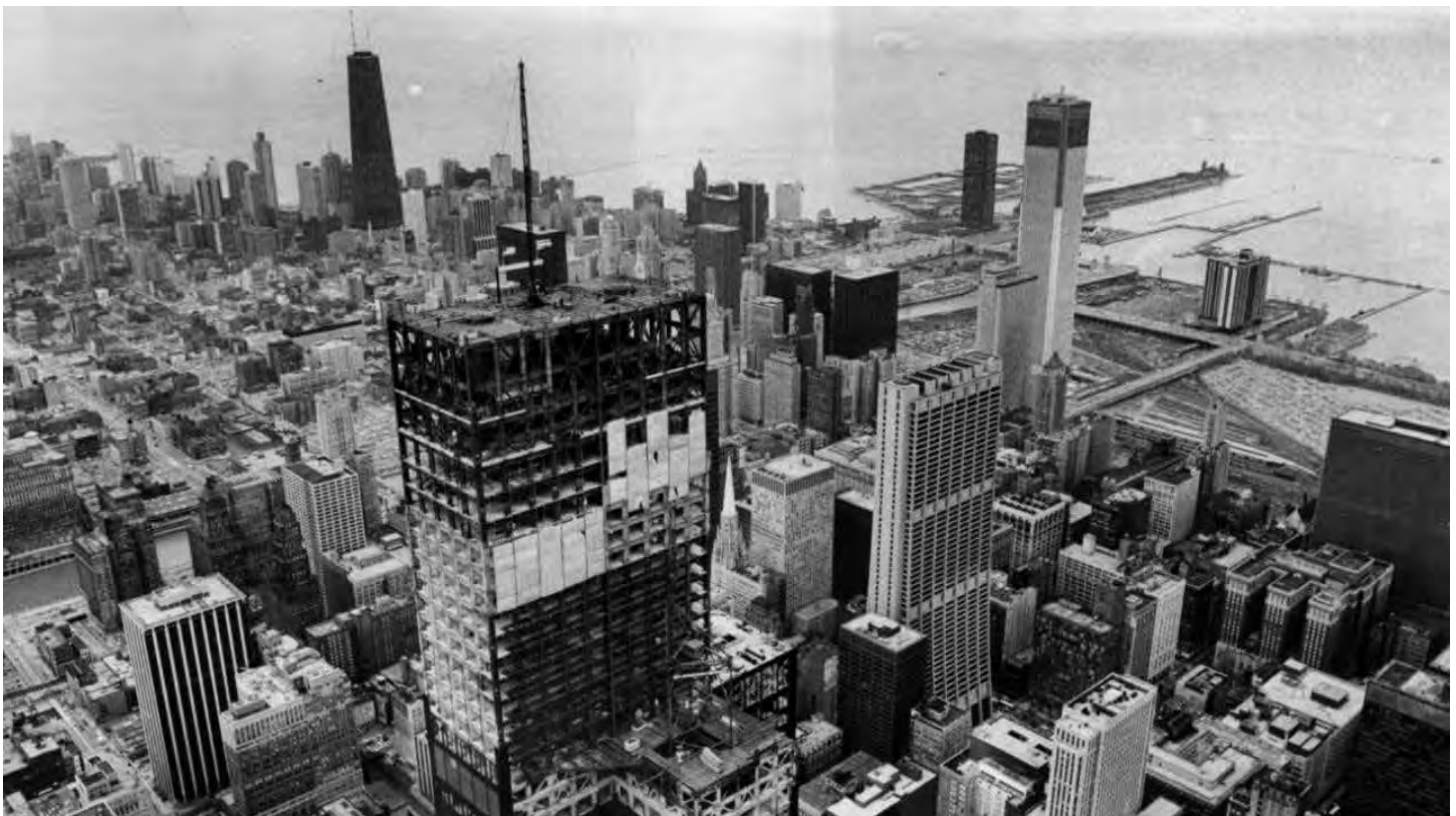
(right) John Hancock Tower; SOM, 1964-69. (below) Sears Tower (SOM, 1969-74) and Standard Oil (Perkins and Will/Edward Durrell Stone, 1972-74) under construction. Both (c) Chicago History Museum.
