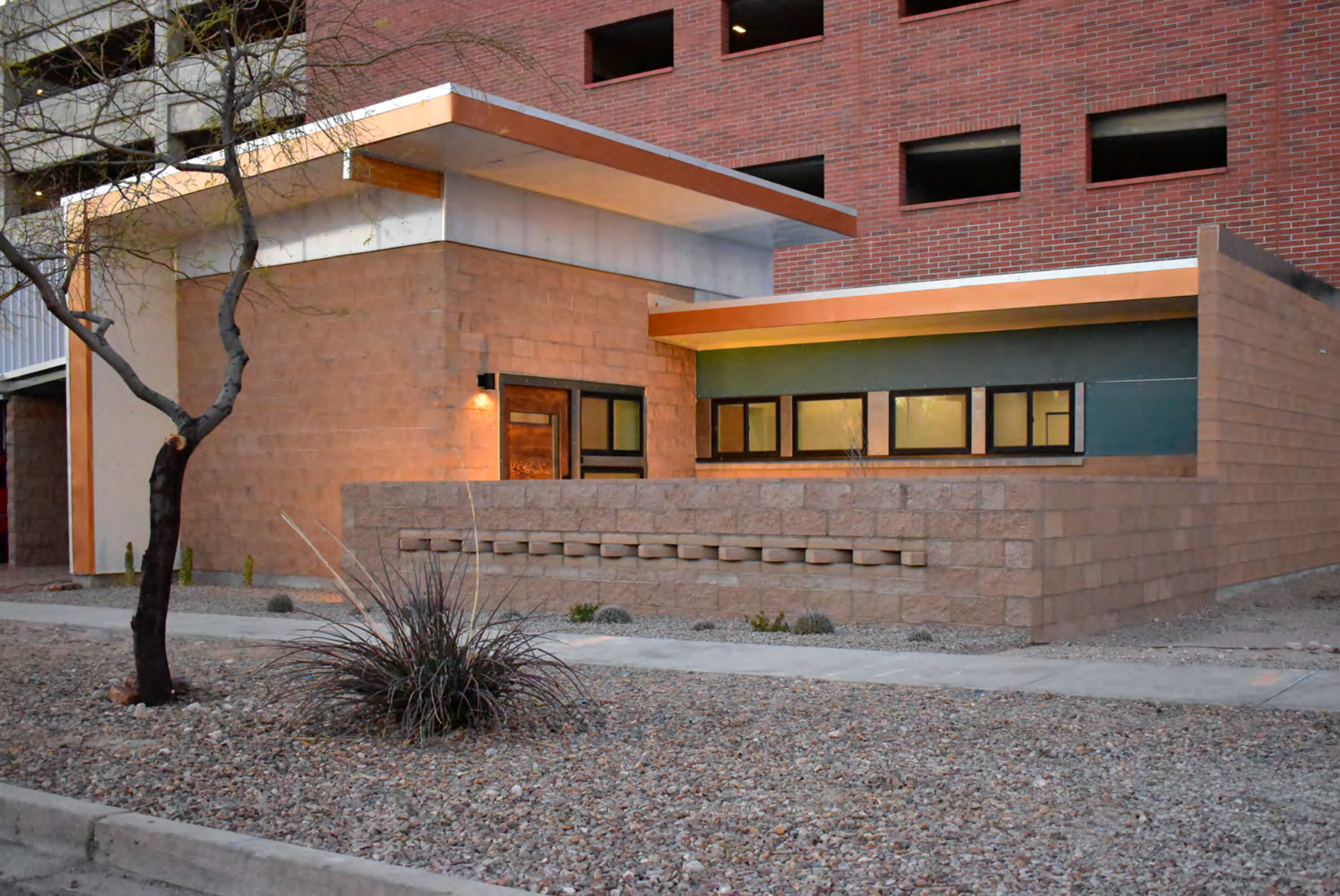
SOUTH STADIUM ROWHOUSE 2
