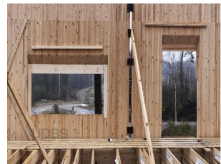
Images of processed dimensional lumber composed into a Wave Layered Timber mass timber structural system, photos, IP, and technology WLT Capital .
