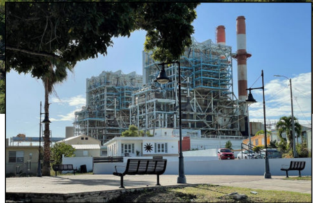
Aguirre Power Station, situated within the Aguirre Community. Photo by Pedro Cruz Cruz
