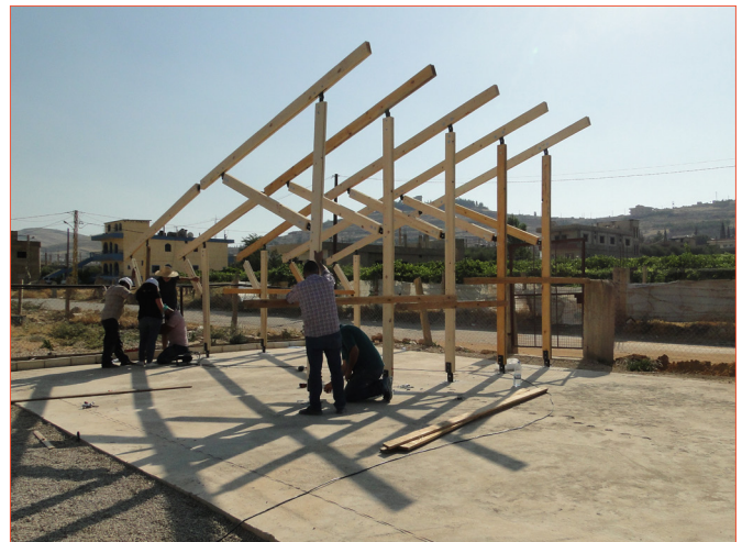
Figure 6. Building the Shams Library in the Bekaa, Lebanon.
