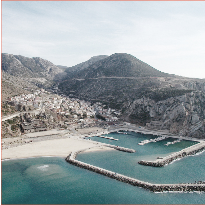
Figure 1. An image of the coastal view of Buggerru. The mining village is set in a narrow and deep valley that opens right to the sea. At both sides of the port (built only recently, in the 90s) are visible the large ruins of the Laveria Malfitano and
