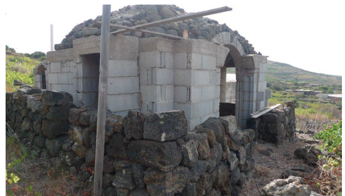
Figure 2. Traditions/contradictions. This typical construction of the islands of Pantelleria and Lampedusa is called dammuso. Originally built in stone and today instead clad in stone.
