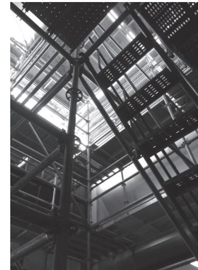
Hospital re-cladding project, KSA. Photo by extern Andrew Cesarz
