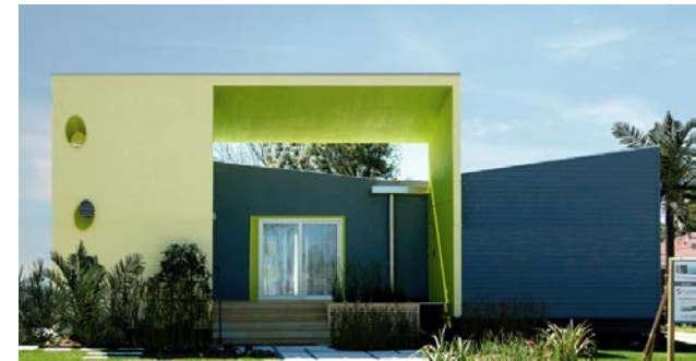
NORTH ELEVATION POST-CONSTRUCTION IMAGE
