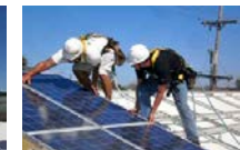
Solar panel installation
