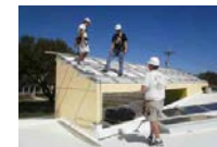
Solar panel installation
