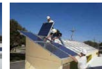
Solar panel installation
