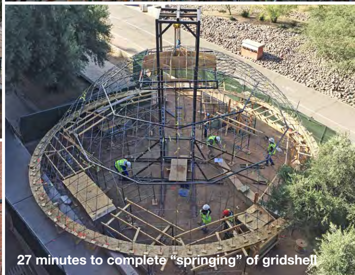
full deployment of suspended formwork
