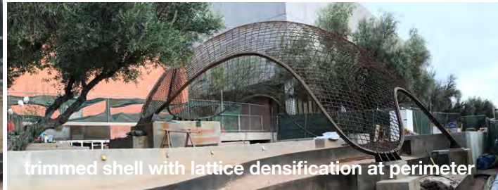
forming and trimming the openings
