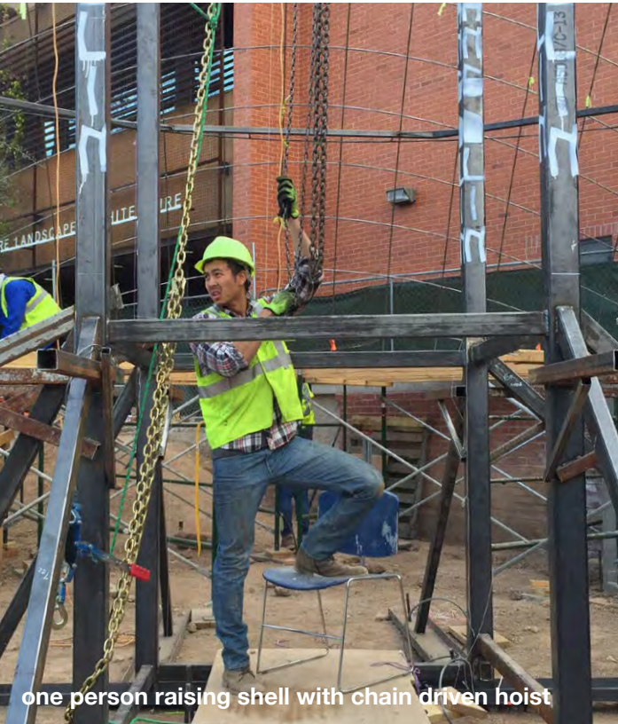
partial deployment of suspended formwork
