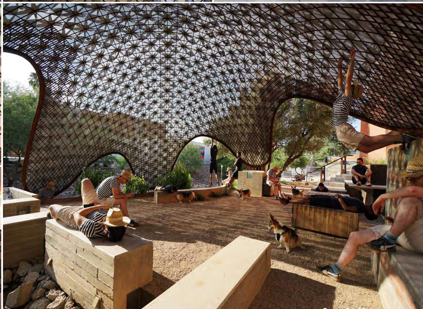
mid afternoon | effects of perforated zinc plated 24 ga. sheet steel shingles
