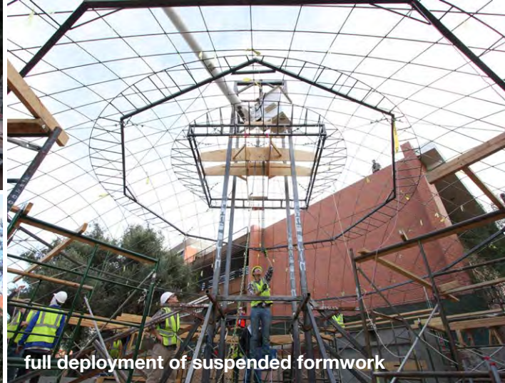
boundary: 37 cold formed and stitch welded 1/2" rods
