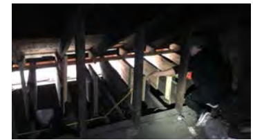
Students collect measurements of existing roof framing.
