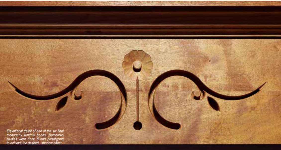
Elevational view of one of the six final mahogany window hoods.
