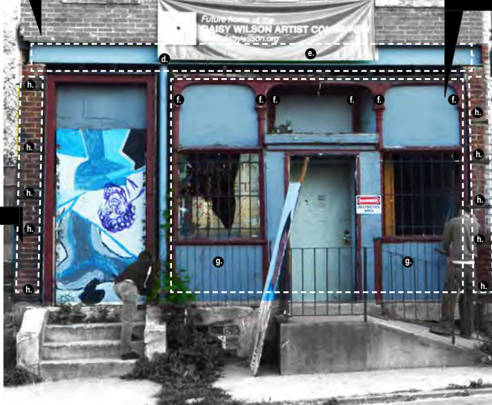
Graphic summarizing research findings and evidence collected by the studio pertaining to each of the missing/damaged components of the building's Bedford Avenue facade. These findings would be used to recreate a historically accurate vision for the facade in Mode 2: VIRTUAL RECONSTRUCTION.
