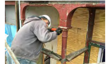
Member of the General Contractor team selectively deconstructs the colonette capital from the storefront in preparation for 3D scanning.
