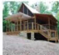
Various overhangs, including trellises, work with the shading system.
