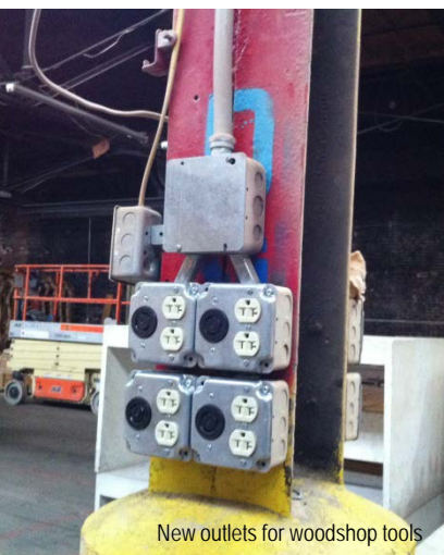
Electrical installation
