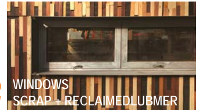
Hopper window reuse in transom Scrap and reclaimed lumber reuse in cladding
