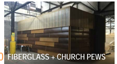
Fiberglass and church pew reuse in tool shed
