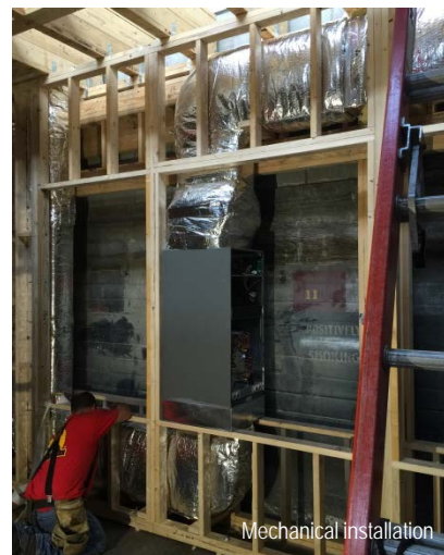
Heat recovery ventilator by city inspector
