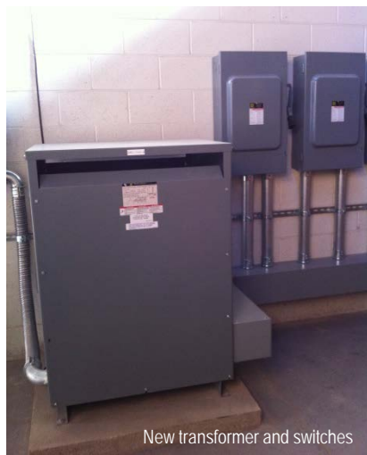
New distribution and power panels
