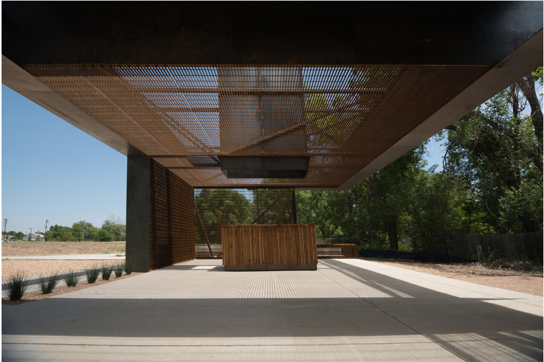
Interior looking at the mobile classroom table. The steel plate on the left wall acts as the shear wall for the structure. The steel oculus helps carry the load of the truss by reinforcing the truss webbing. Lakewood Gulch, and the future Lakewood Gulch River Trail, are on the right.
