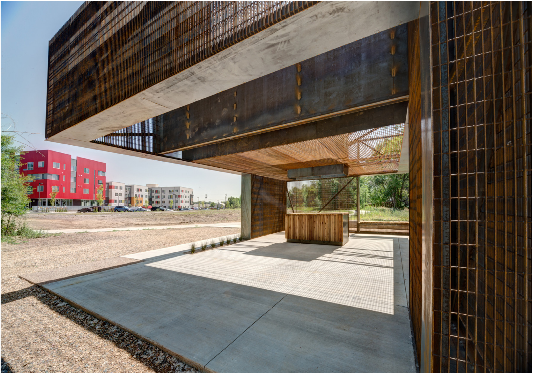
Looking northeast through the cantilever. The Metro West Housing development is in the background .
