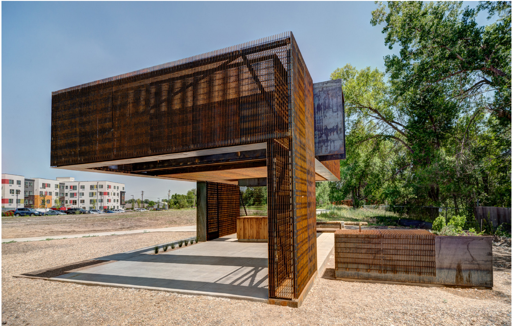
Looking northeast. The "entry gutter" drains into the wash station. The water from both drain into the herb garden watering the herbs throughout the year. The core ten bridge to the Head Start program can be seen in the distance.
