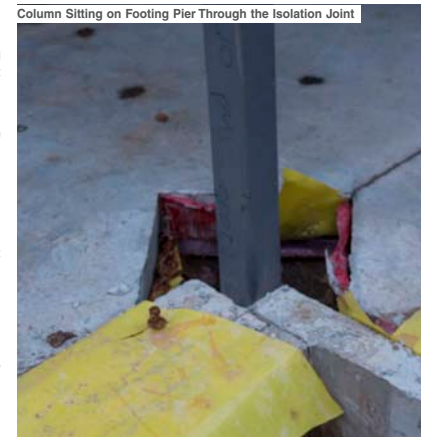
S4.3 Plan of Column Isolation Joint
