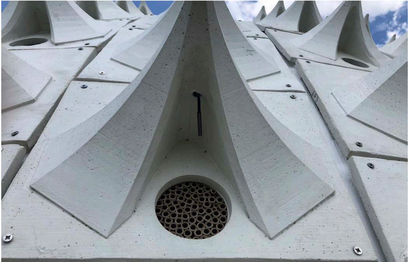
Figure 4. Ductal panel with cardboard nesting tubes and endoscopic camera, Pollinators Pavilion, Harrison Atelier, 2020..
