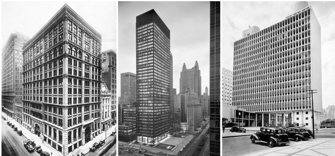
Figure 1. Home Insurance Building, Le Baron Jenney, Chicago, 1885. Seagram Building, Mies van der Rohe, New York, 1958. Ministry of Education and Health, Lucio da Costa, Oscar Niemeyer, Affonso E. Reidy, et al. Rio de Janeiro, 1945. Evolution of the façades according to modernist canon; note the different approach in the Seagram and in the prescient critically regionalist Brazilian architecture despite the time of completion.
