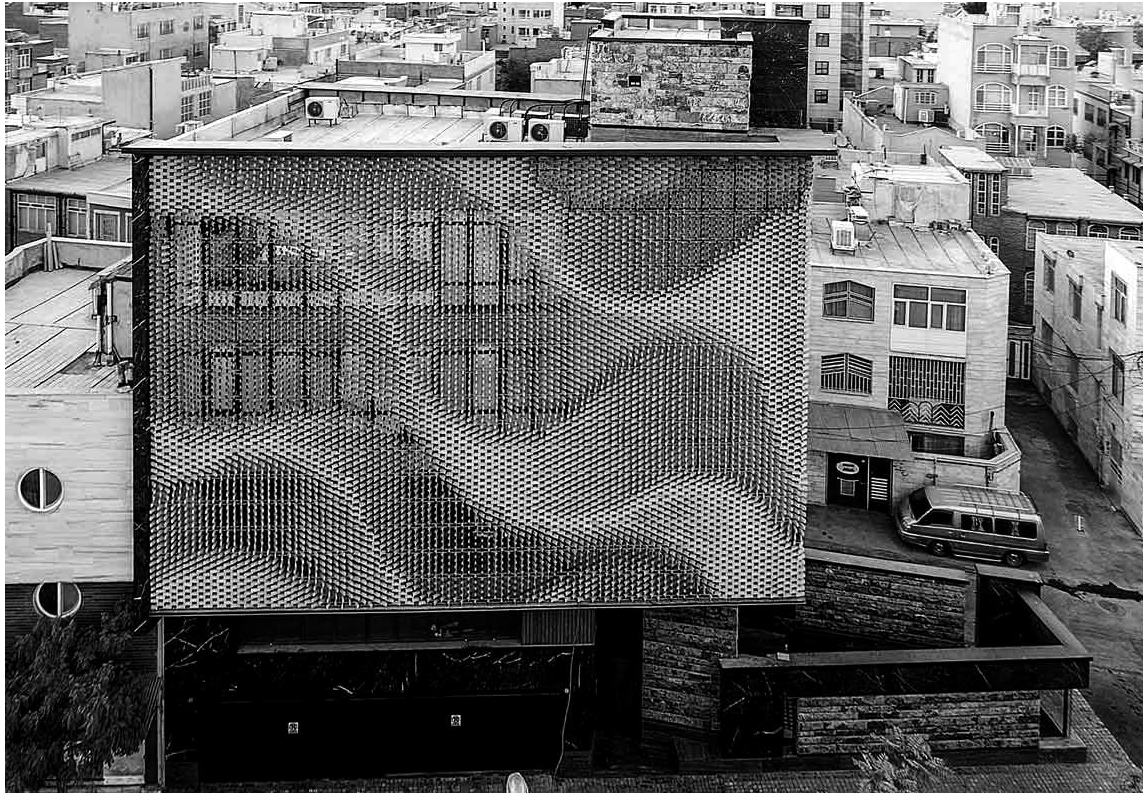
Figure 3. Latticed revolving bricks façade, Farhad Mirzaei in Arak, 2015.
