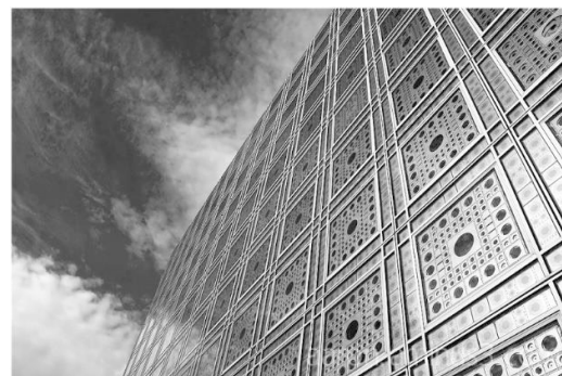
Figure 2. Institut du monde arabe. Jean Nouvel, Paris. 1985. One of the first examples of kinetic façades.
