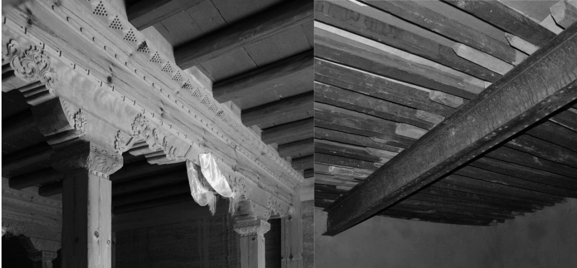
Figure 3. A Tibetans Shrine Traditionally Constructed and a Steel Beam in an Auxiliary Room. Photograph by Author
