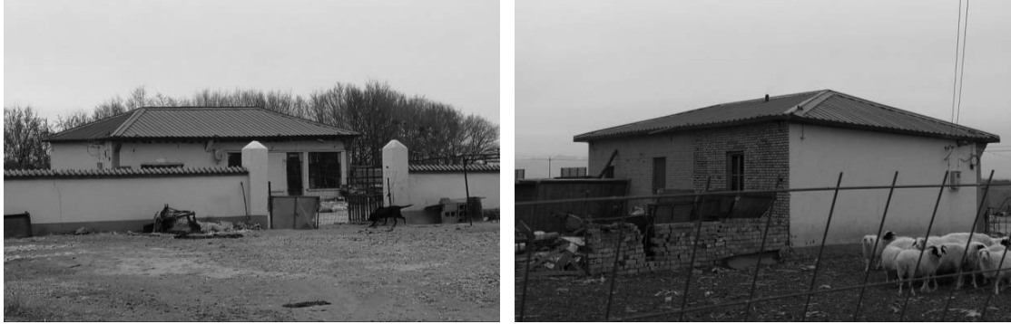
Figure 3. the process of renovation; the renovated houses
