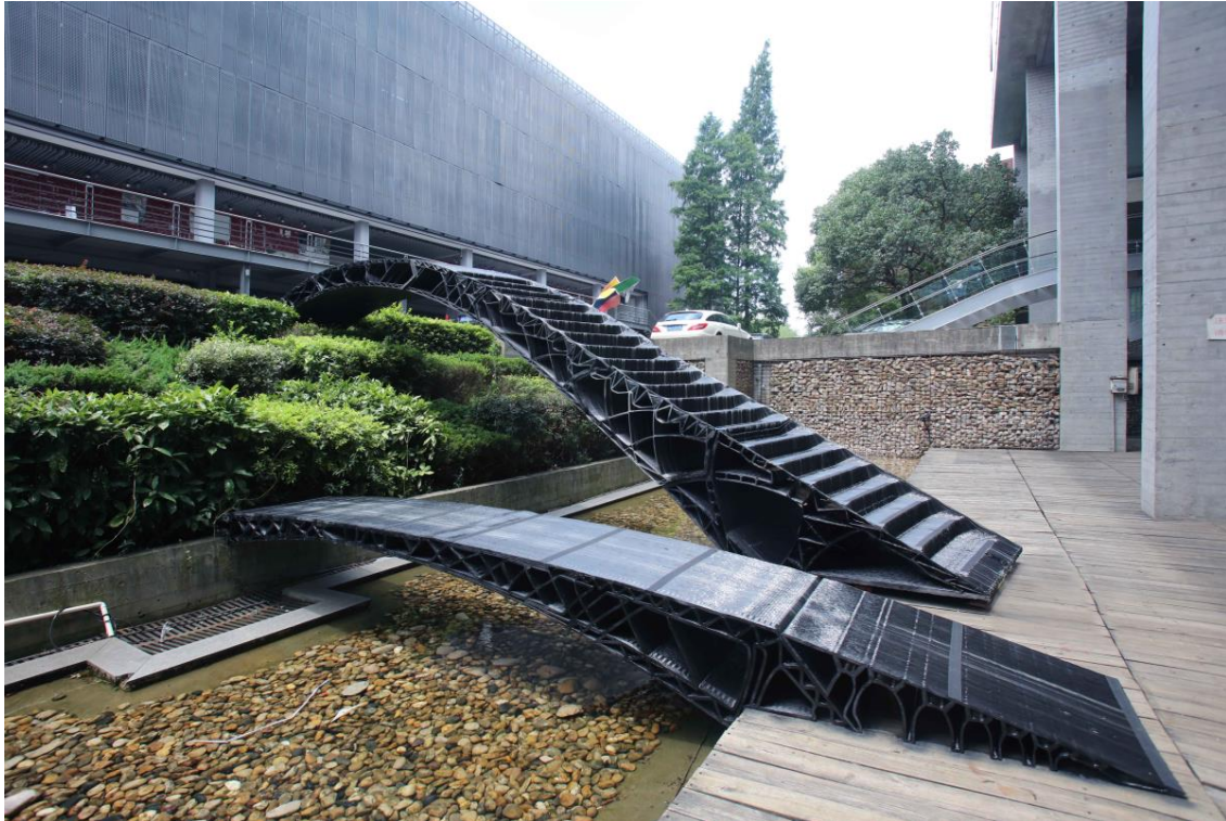
Figure 3. 3D Printed (Modified Plastics) Footbridge in Tongji University by DDRC&FabUnion in 2017.
