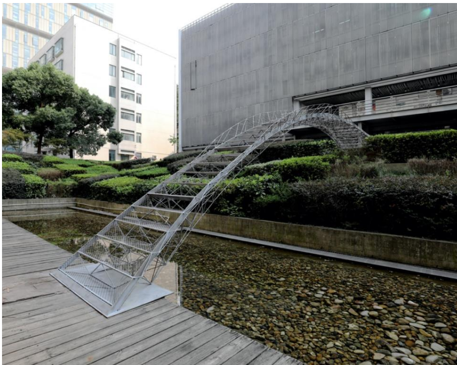
Figure 4. Printed(Metal) Footbridge in Tongji University by DDRC&FabUnion in 2018.
