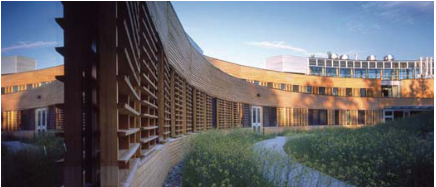
Figure 3: Perkins + Will with Alfred Waugh, Nicola Valley Institute of Technology, University College of the Cariboo.
