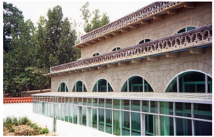
Figure 4 : A modernized “cave dwelling” in Western China using compressed earth blocks and passive solar design for improved interior comfort and reduced fossil fuel use.
