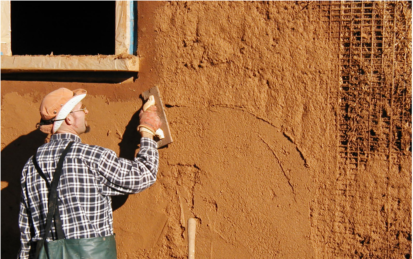
Figure 3: Applying earthen plaster to a strawbale winery in Healdsburg, California. This winery keeps wine and people naturally cool. Photo credit: Joseph F. Kennedy.
