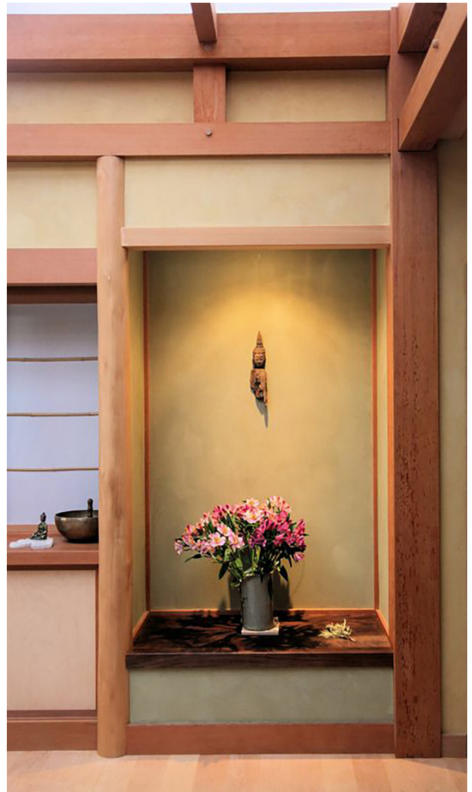
Figure 1: A salutogenic house – timber frame with light-clay insulation, plastered with earth plaster and finished with natural paint. Photo credit: Paula Baker-Laporte.
