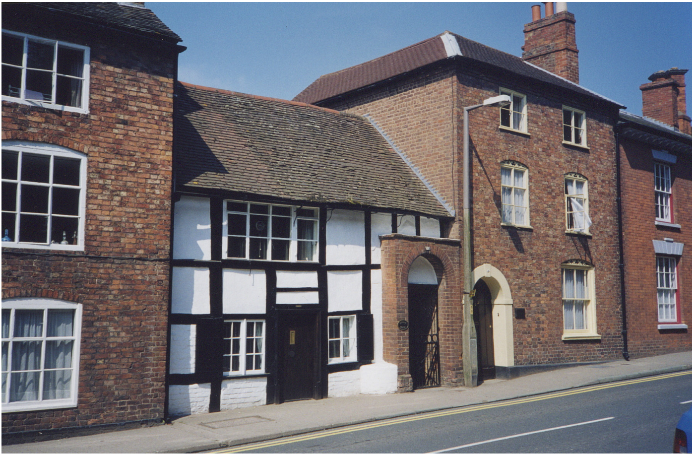
Figure 2: A several-hundred-year-old traditional timber frame house with wattle and daub infill in a northern European city. Photo credit: Catherine Wanek.
