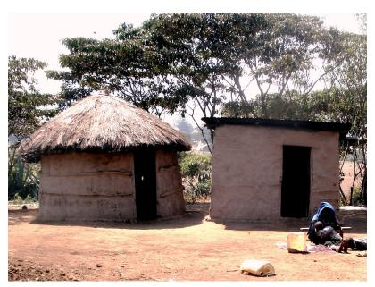
Figure 2: Typical Wattle and Daub construction at a compound in Musa. Here also illustrates an example of both a thatch roof (left) and corrugated metal roof (right) (Reineccius 2012).
