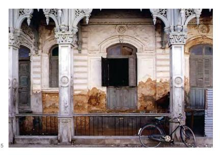
Figure 5: Unlike lime plaster, the Portland cement is not compatible with the masonry substrate, leading to water damage to the structural walls. (Aga Khan Trust for Culture 1993).
