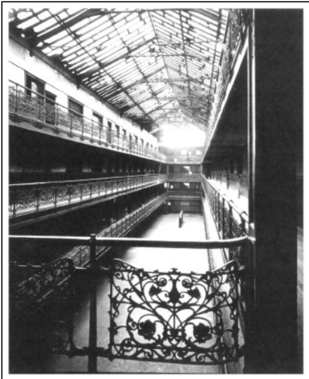
Figure #3: Mecca Flats Covered Court
