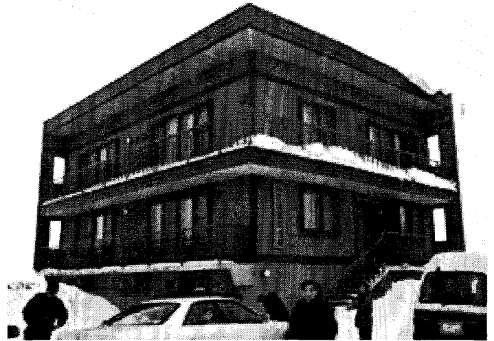
Fig. 1. Early large KST house design, possibly 'Elm' model. Note the monolithic concrete base, balconies and wind breaks.
