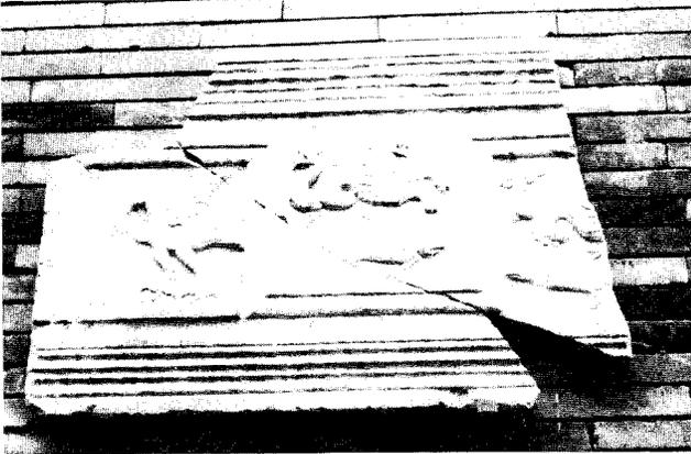
Fig. 8 Typical Roman artifact displayed on the background of an abstract brick plane. The taught surface of the brick is achieved by the use of frogs for the mortar.
