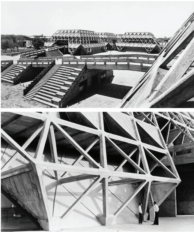
Figure 4. Halls of Industries, exterior; exterior close-up view of cast-in-situ structural joints. University of Chicago Press, 2016.
