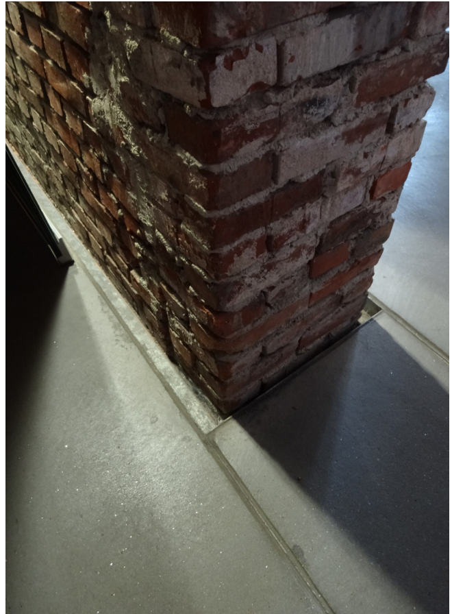
Figure 3: Raw wall and finished floor. Photo by Author.
