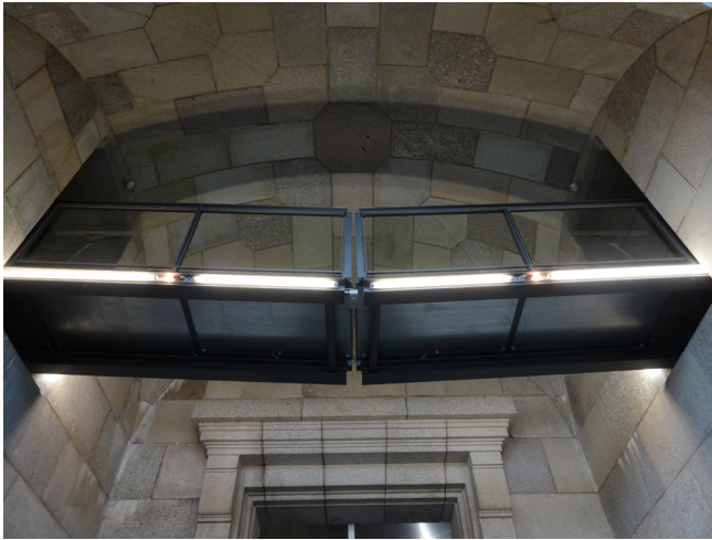
Figure 2: View of the Bridge. Photo by Author.
