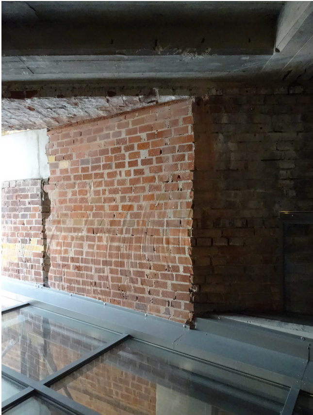
Figure 5: The physical trace of the circular saw is visible in the brick wall. Photo by Author.
