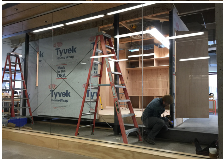
Client and engineering review, CNC fabrication and Mock-up
