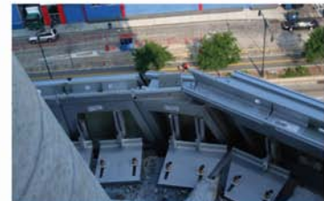
01 Overall view, west facade 02 Embeds / brackets supporting panels 03 Curved fitting / connection between panels
